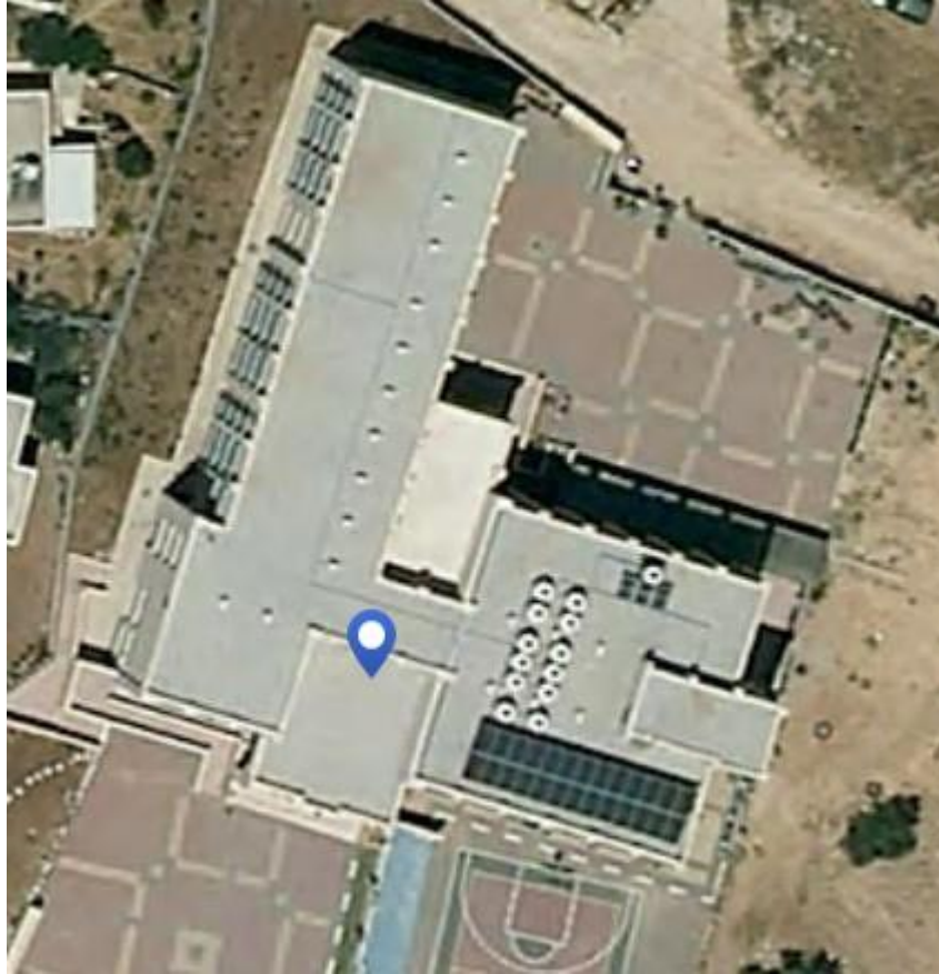
Fig. (2.8): Al-sakra primary school
