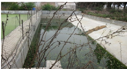
Photo (2): the first pool using for wastewater treatment by Duckweed
