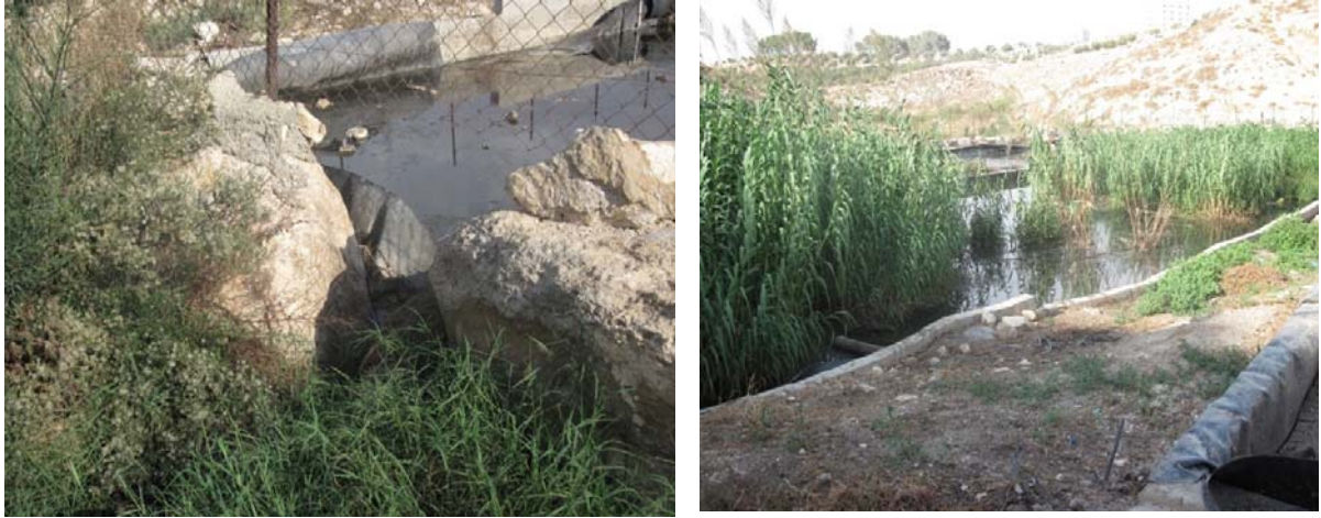
Photo (5): Nuba WWTP
