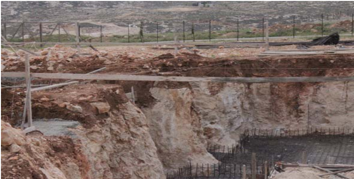
Appendix 5.6: Excavation in site showing soil strata.(25/3/2010)
