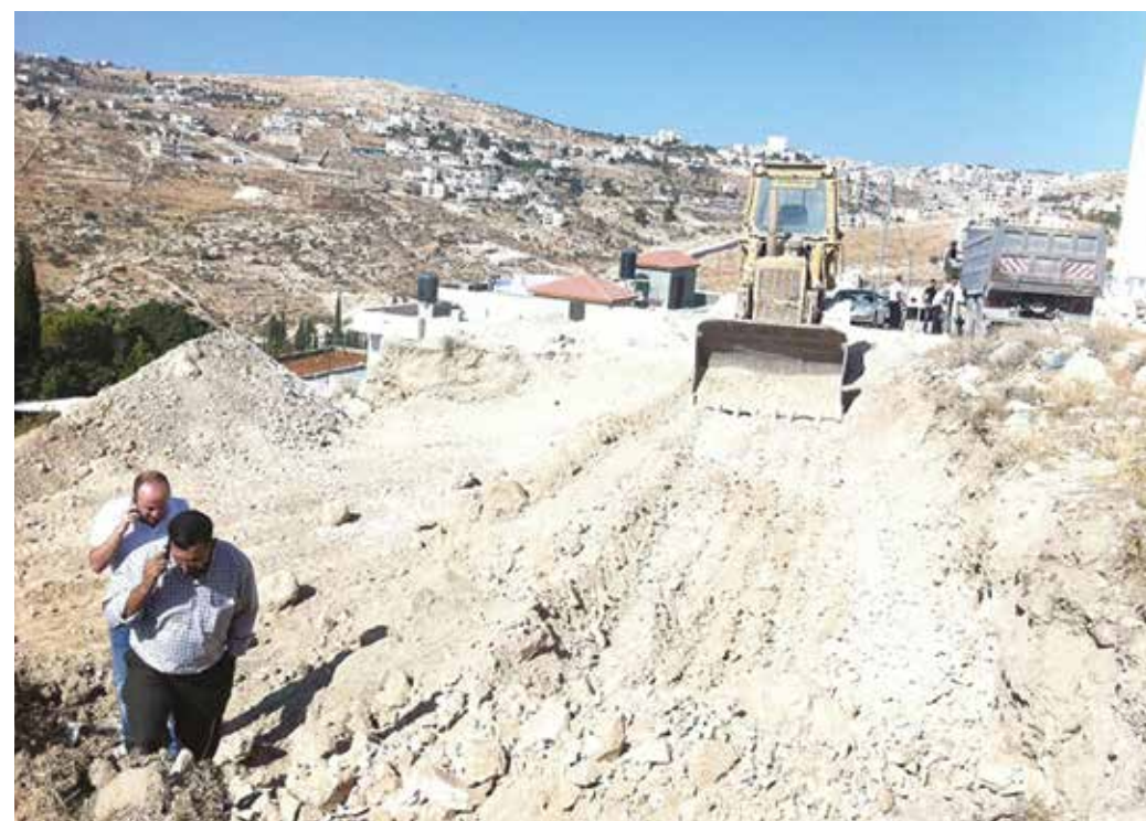
Figure 4. External wall destruction by a bulldozer. Photograph by the author.
