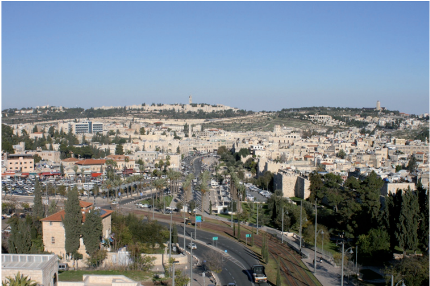
Junction between Sultan Sulaiman Road and Road number 1
