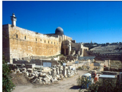
Figure (9): Plan and photo of the Umayyad Palace and its auxiliary buildings.
