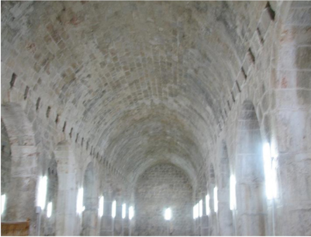
Figure (8): Solomon’s Stables, barrel vault roof and piers.
