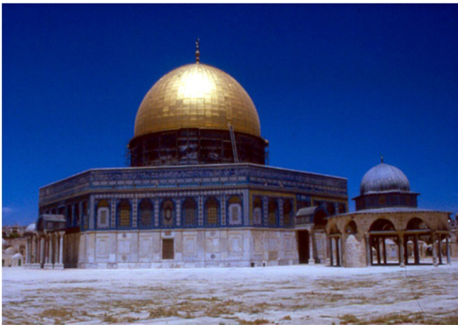
Figure (4): General view of the Dome of the Rock
