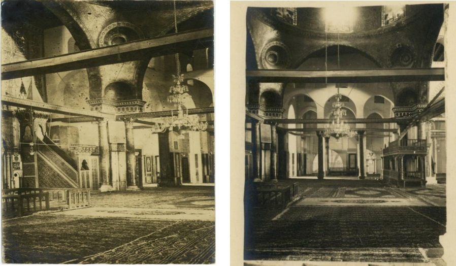
Figure 9: The reconstruction carried out under the supervision of Kamal Al-Din in Al-Qibli Mosque.
