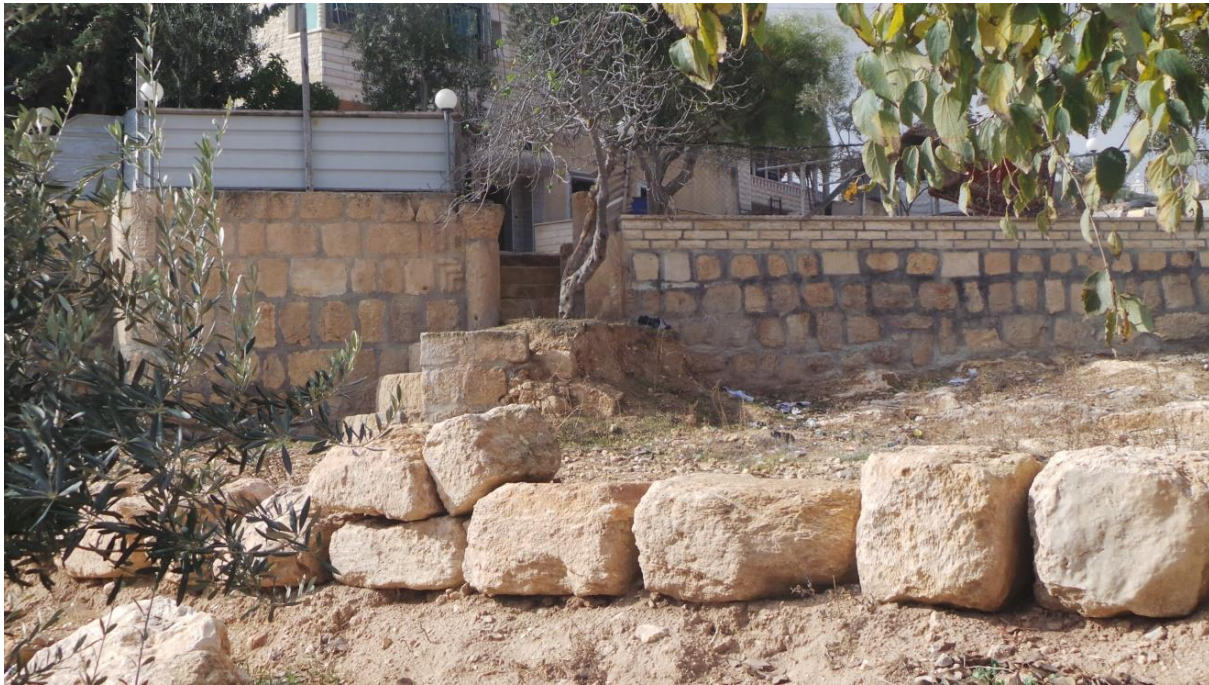
Figure (22), a traditional house constructed by the old stones (re-usable) from the archeological site (the castle), 2019.
