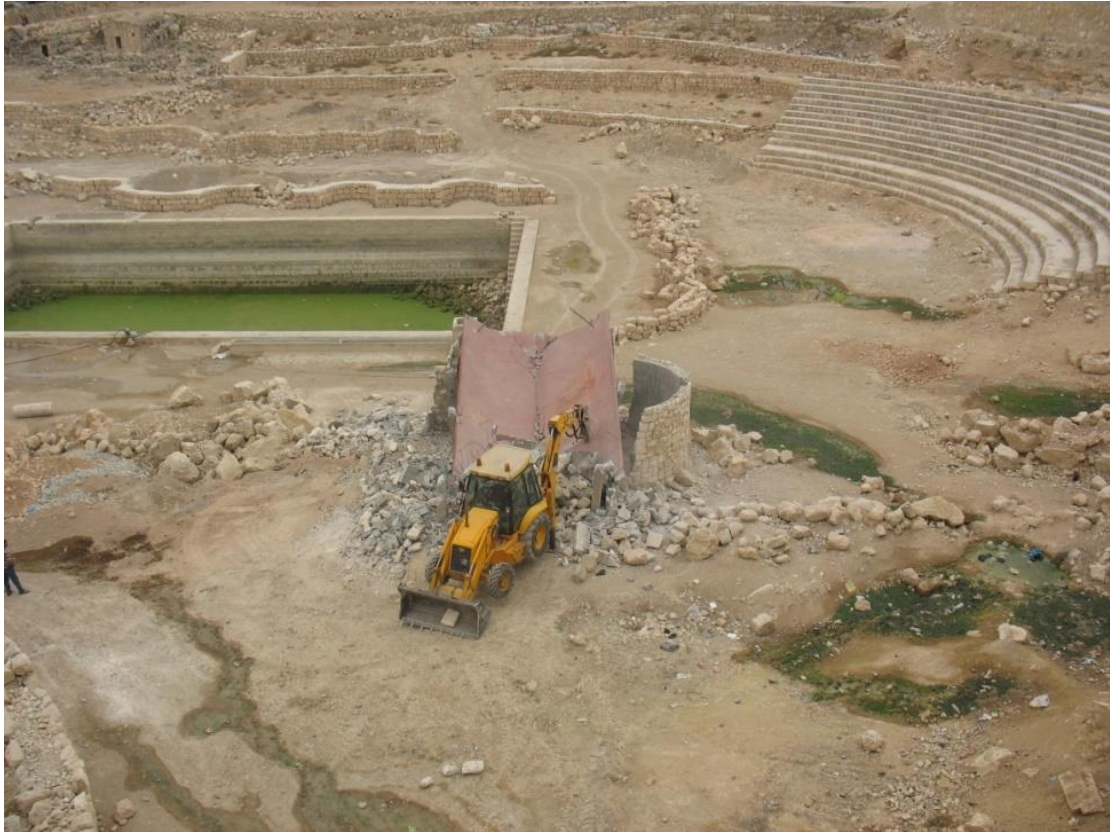
Figure (11): Al-Karmil's Pond during rehabilitation (The Achieve of Yatta Municipality).
