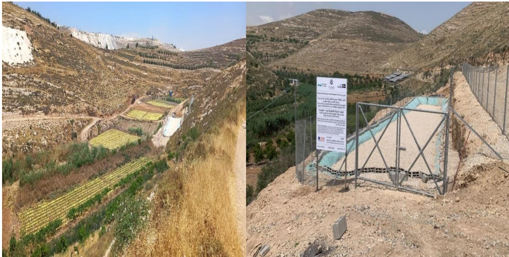
Figure 7: Sear (Al-Aroub) WWTP as post-treatment for Secondary treated WW from Arroub camp.
