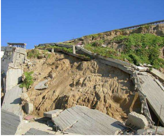
The Current situation of the site
