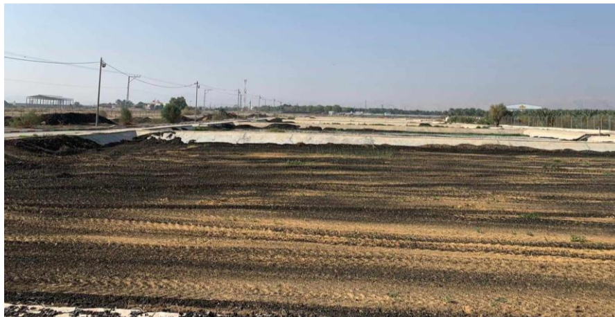
Figure 3.3: The drying beds of the sludge at JWWTP
