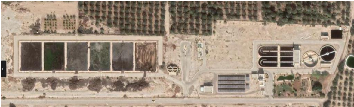
Figure 3.2: The Jericho Wastewater Treatment Plant (Google Earth, 2022)
