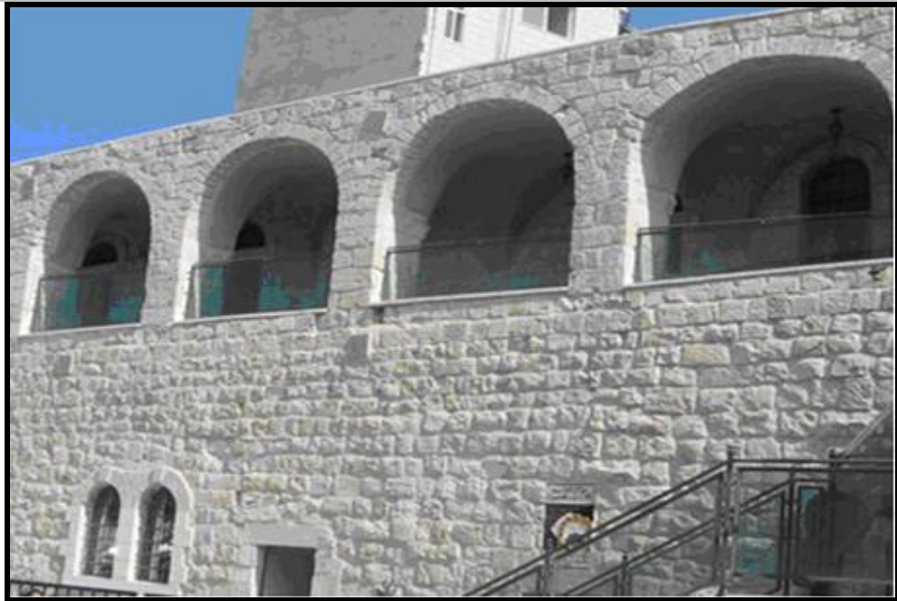
Figure (5.16): The Ottoman Court Building After Rehabilitation Source: Researcher
