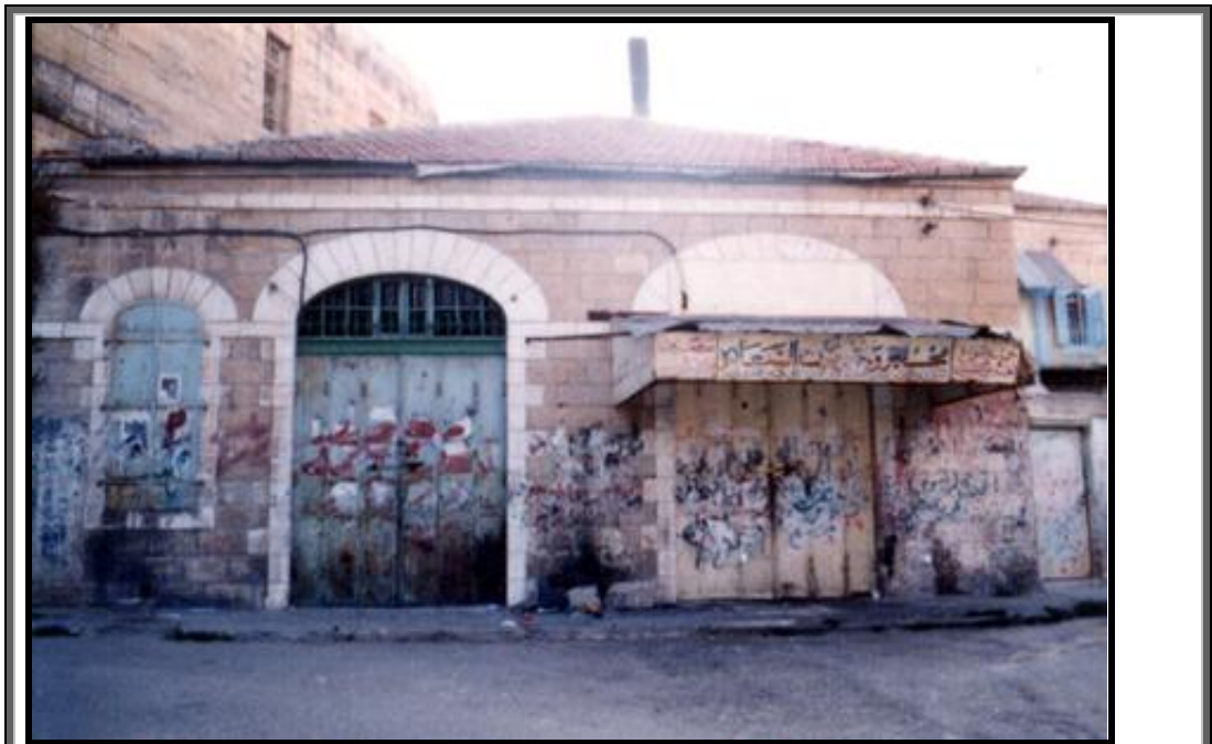
Figure (5.14): Hanania Commercial Stores, Ramallah. Source: Al-Juabeh and Bsharah, Ramallah Architecture and History (2002)
