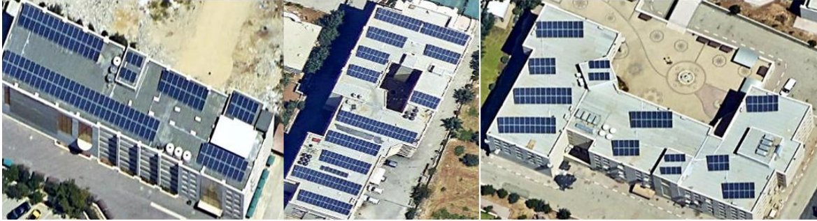
Figure 3.28: Satellite photo of the PPU PV System.
