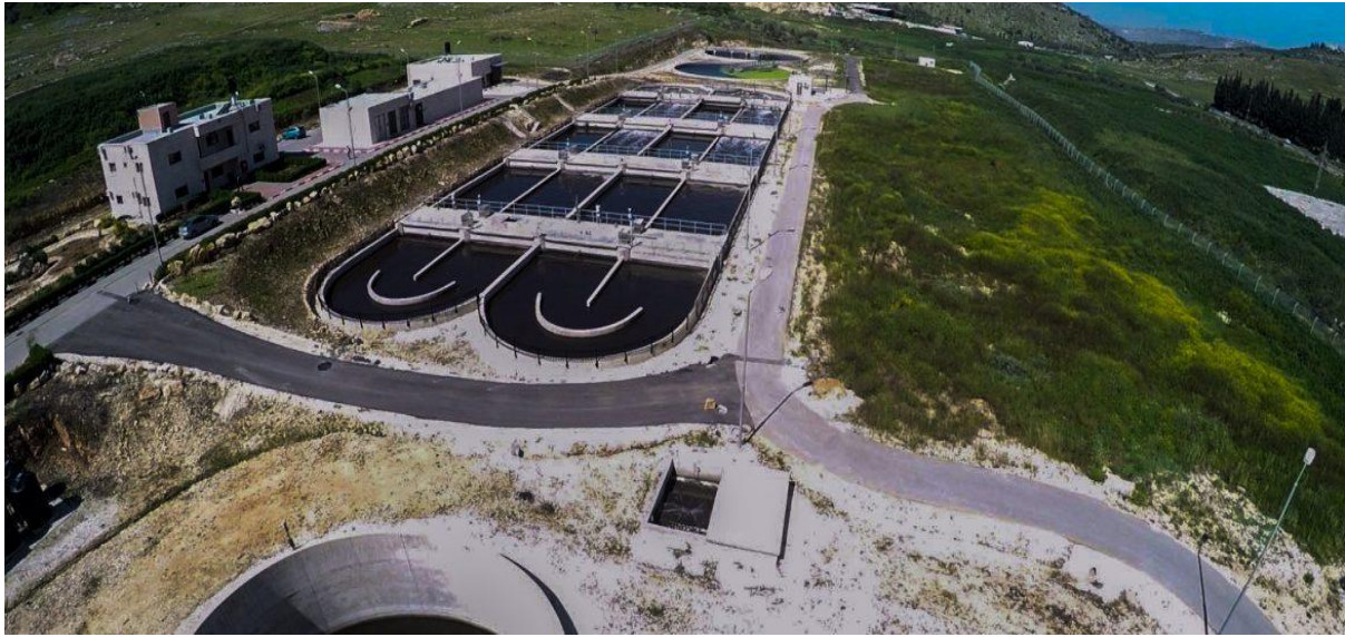
Figure 11: Nablus West WWTP (wwtp.nablus.org)
