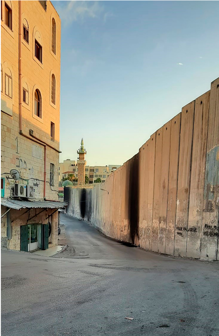
Figure 4. Kuba Junction, the Abu Deis-Ezariyah side of the Segregation Wall.
