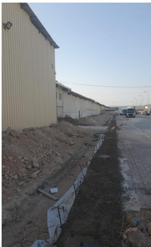
Figure 9: The dead space on the side of factory buildings
