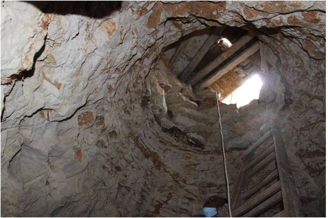
Fig. 4: The mouth and covering materials of the septic tank, looking upward. Photo by the authors.
