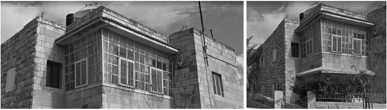
Fig 6. A typical Baranda covered with tilted iron frames and glass.
