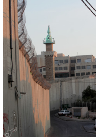
Separation Wall at Ras Kubsa Junction
