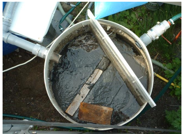
Photo A8: Excessive sludge accumulated in ST.
