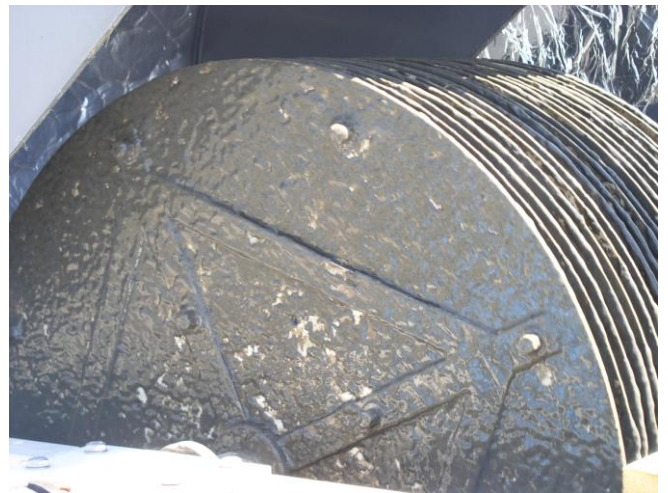
Photo A4: Biofilm attached on rotating discs
