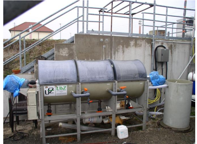
Photo A2: RBC after its first installation.
